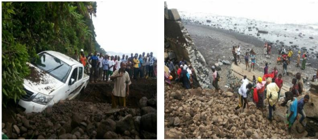
Fig. 8 Coastal erosion processes along a Comorian shoreline and their impacts on road infrastructure
