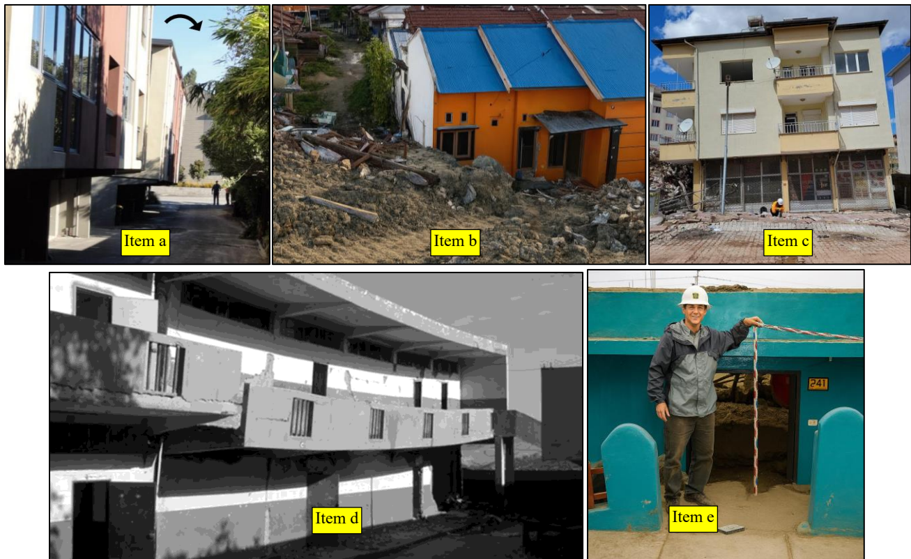
Fig. 1 Cases of soil liquefaction
